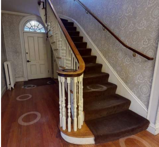
Figure 8: Main staircase handrail.
