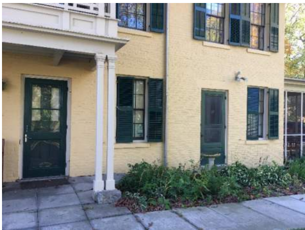
Figure 6: Accessible entrance and door at east elevation.
