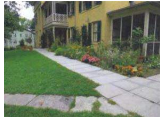
Figure 5: Accessible walk at east elevation.
