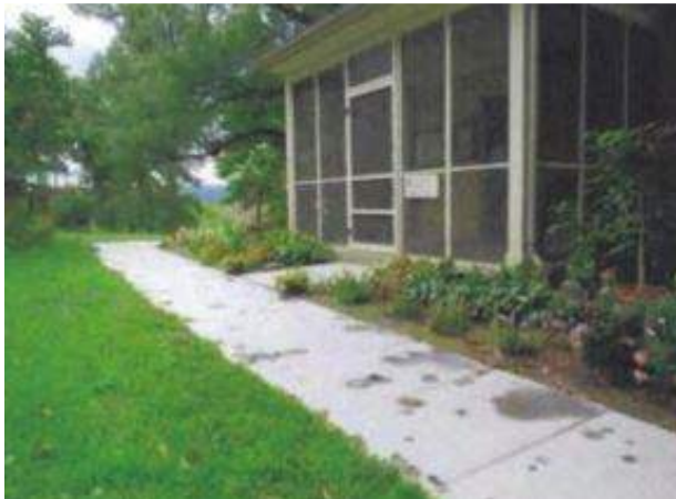
Figure 4: Accessible walk at north elevation.
