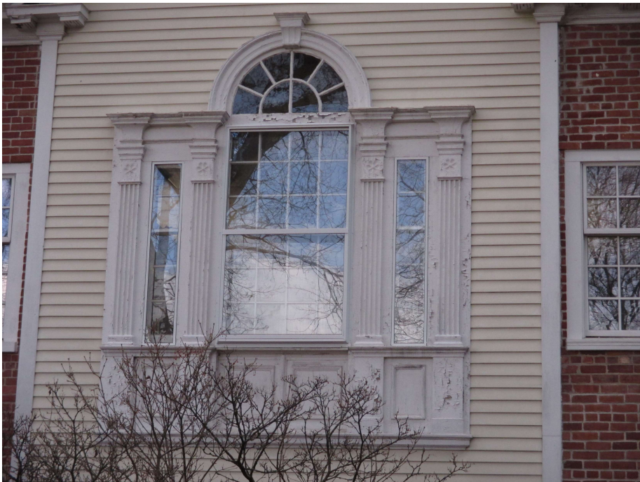
19. North elevation, second floor window detail, view south
