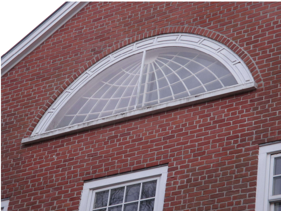
23. North elevation, upper floor window detail, view southeast
