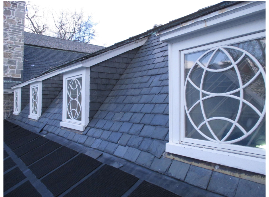
172. Roof level, view northeast
