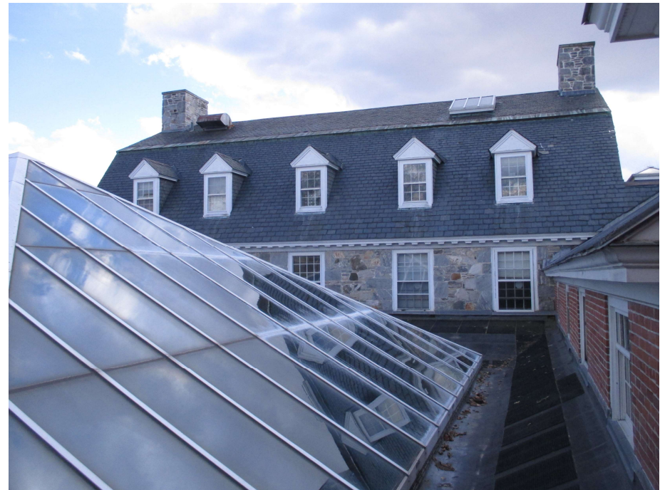
168. Roof level, view south
