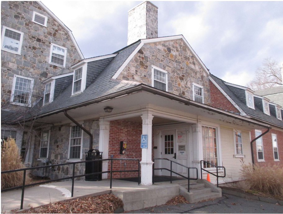
5. South elevation (left) and east elevation (right) of east wing and primary active entrance, view northwest
