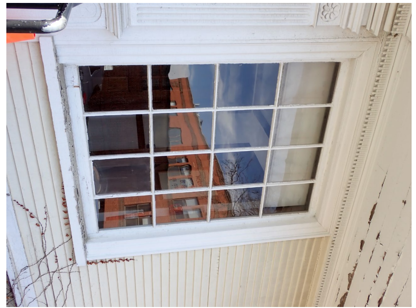
2. East elevation, first floor, typical historic fixed wood window
