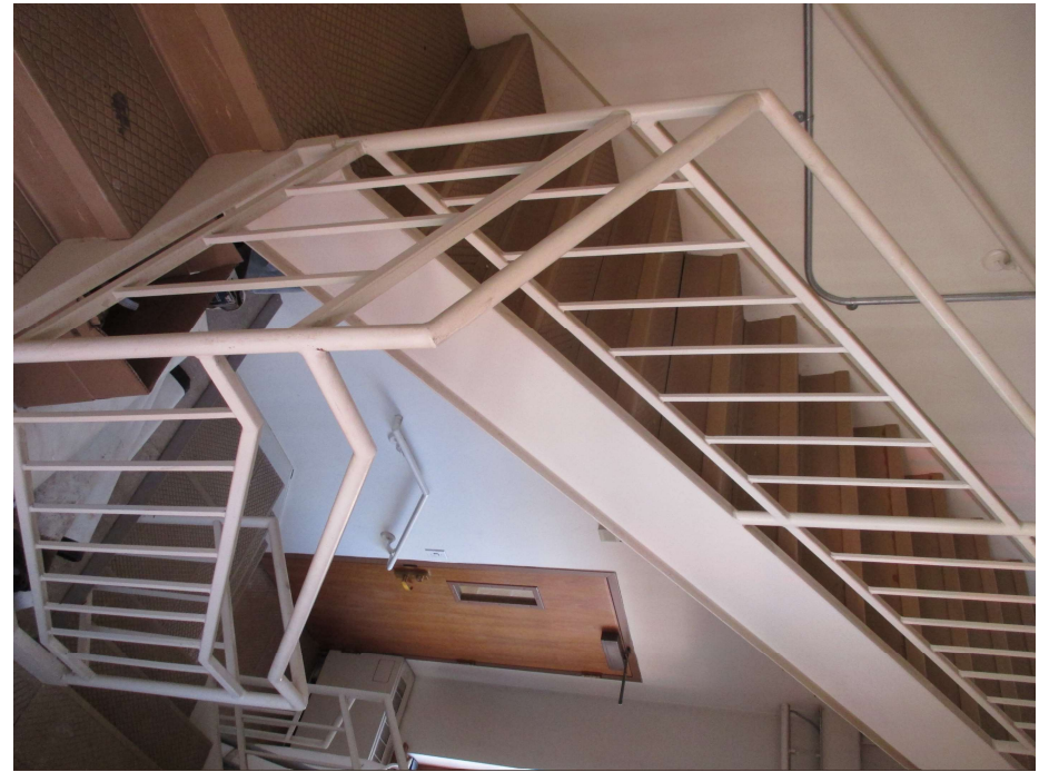
62. Lower level, northeast stair, view northwest
