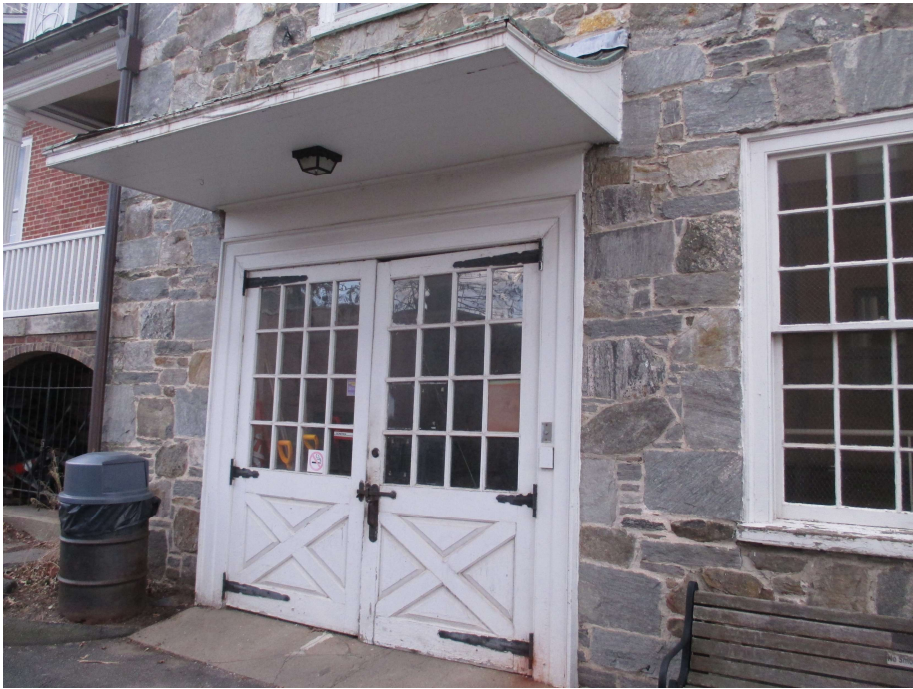
29. East elevation, ground level entrance, view southwest
