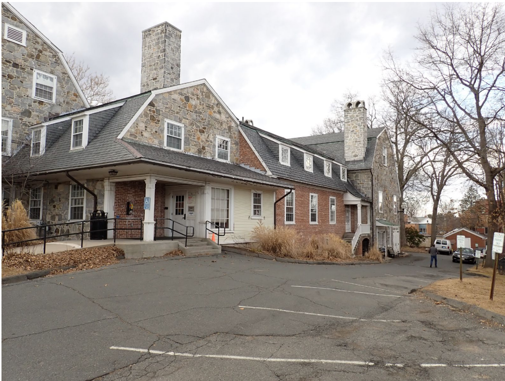
2. East elevation, view northwest
