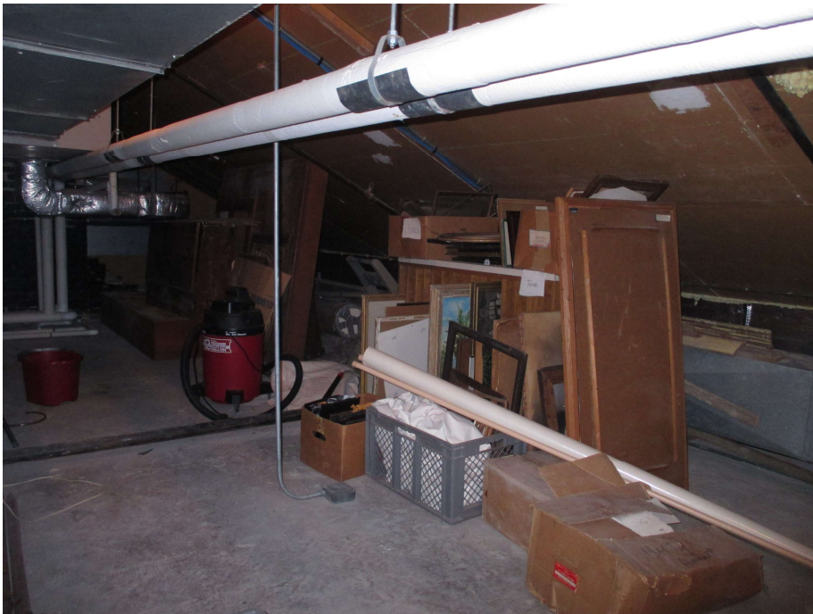
167. Attic level, view southeast
