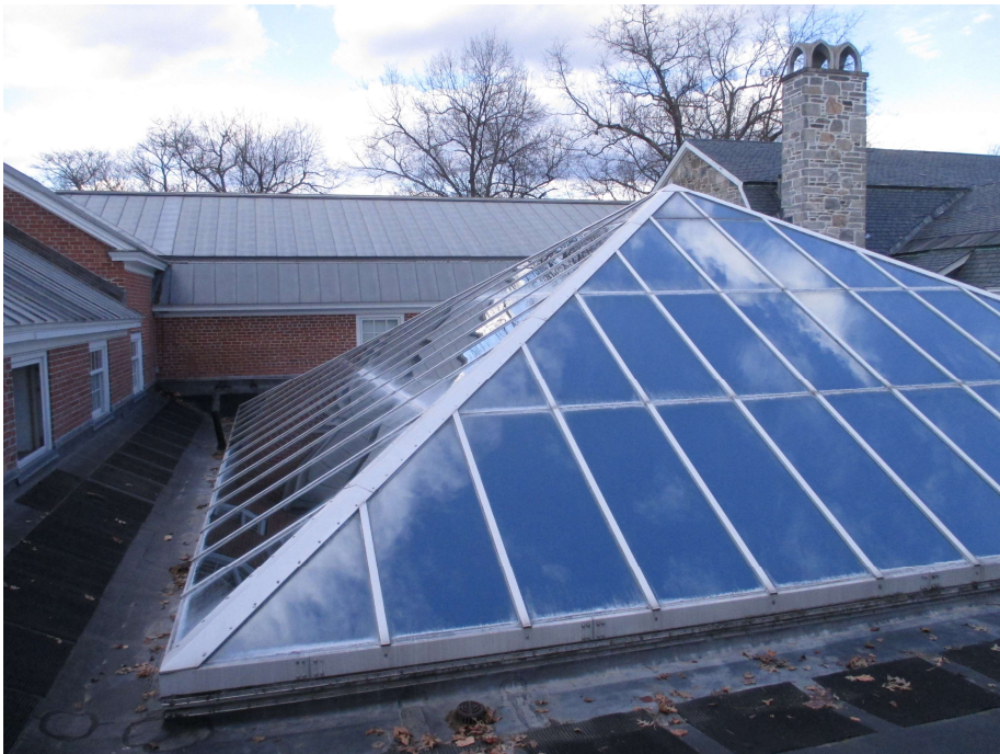
175. Roof level, view north
