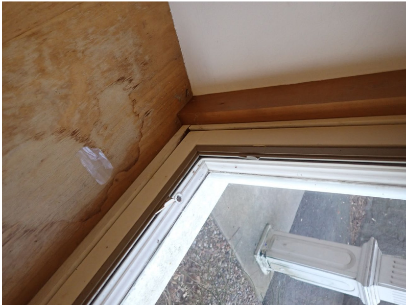
15. Basement level, north wall, detail of typical 1993 double-hung wood window condition
