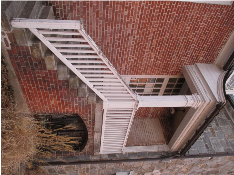
27. East elevation, secondary entrance, view northwest
