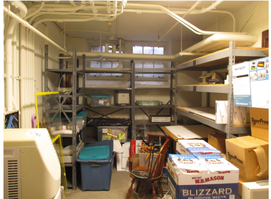
32. Lower level, storage closet, view east
