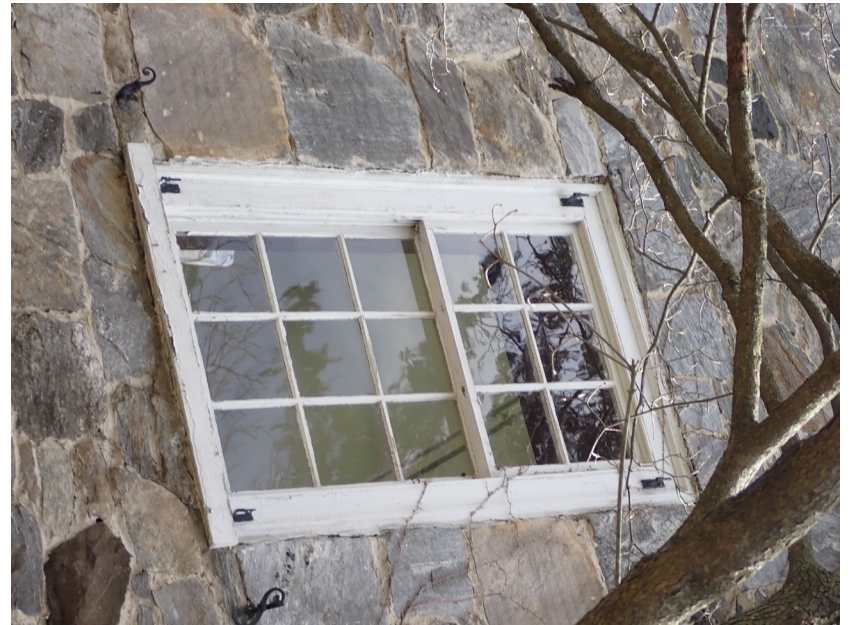
4. West elevation, second floor, typical historic double-hung wood window
