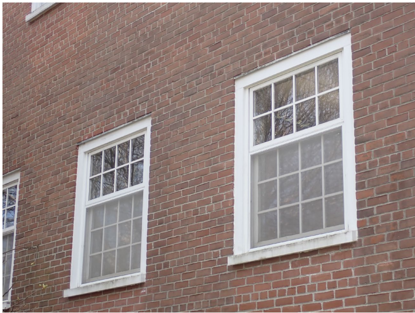
9. North elevation, second floor, typical wood windows at 1993 addition
