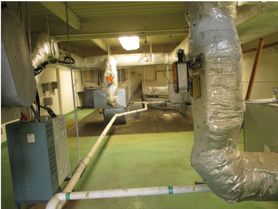
163. Third floor, mechanical room, view west
