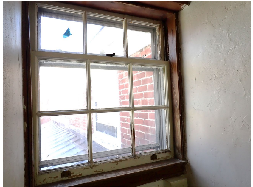
50. Second floor, west wall, typical historic double-hung wood window
