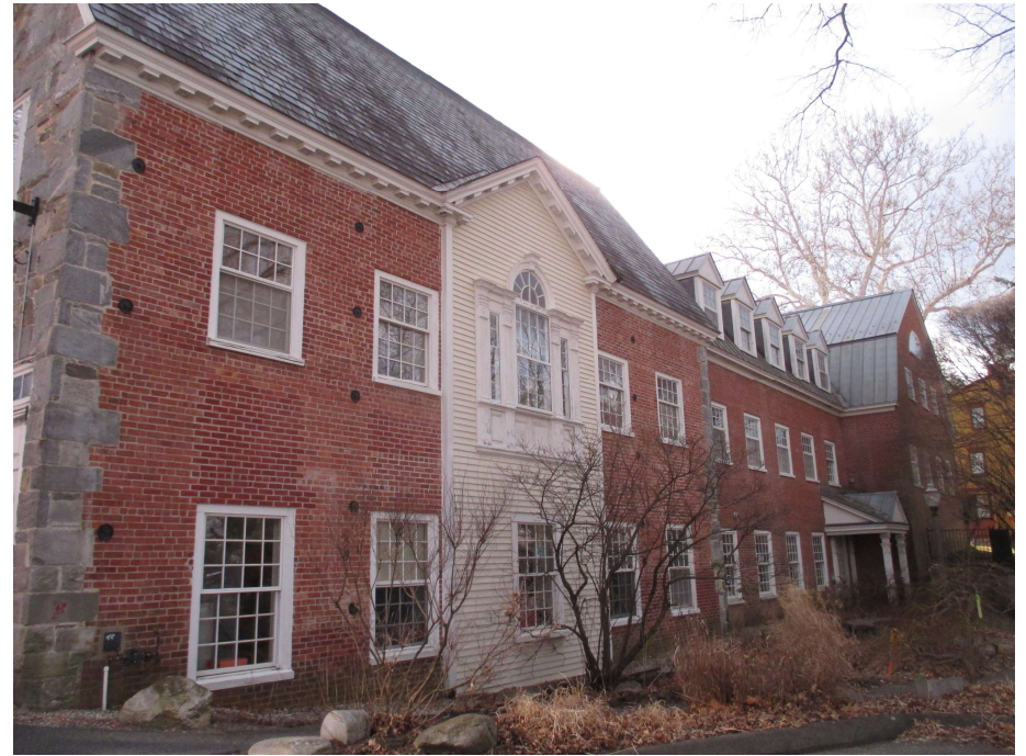
18. North elevation, view southwest
