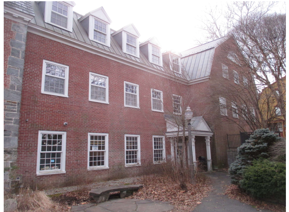
20. North elevation, view southwest
