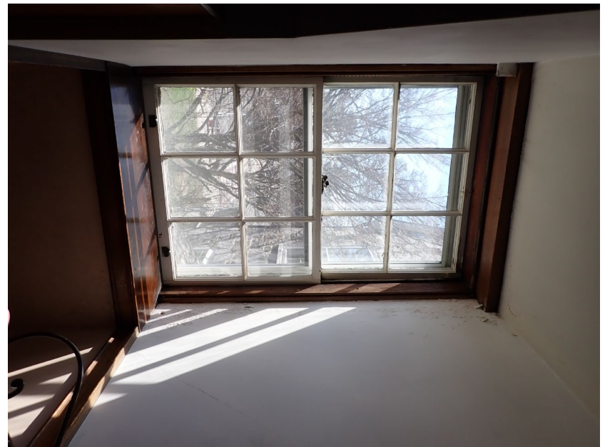
38. Second floor, south wall, typical historic double-hung wood dormer window
