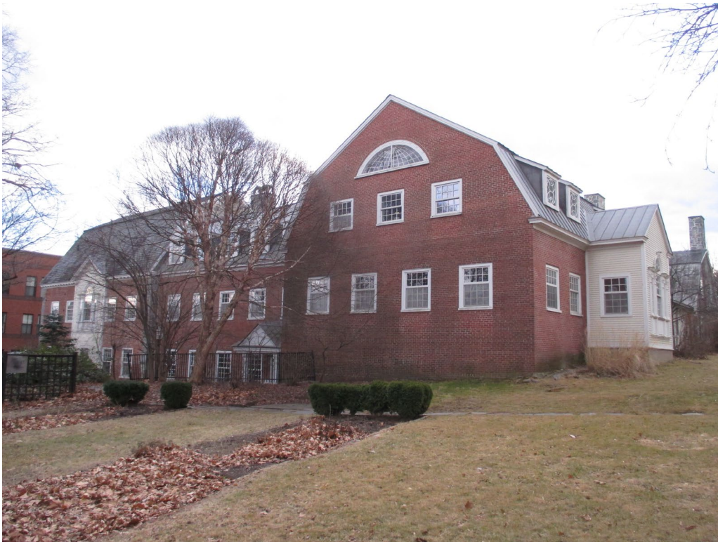
4. North elevation, view southeast
