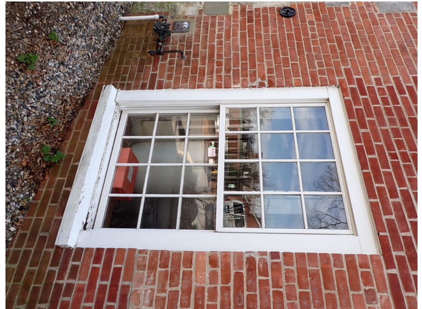
8. North elevation, basement level, typical replacement wood window
