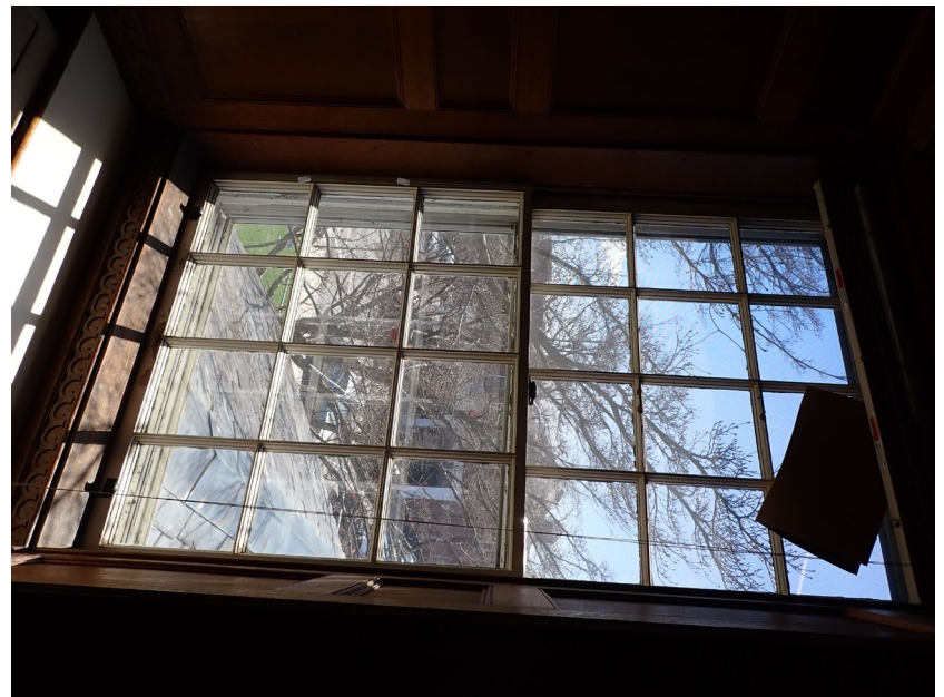
42. Second floor, south wall, typical historic double-hung wood window
