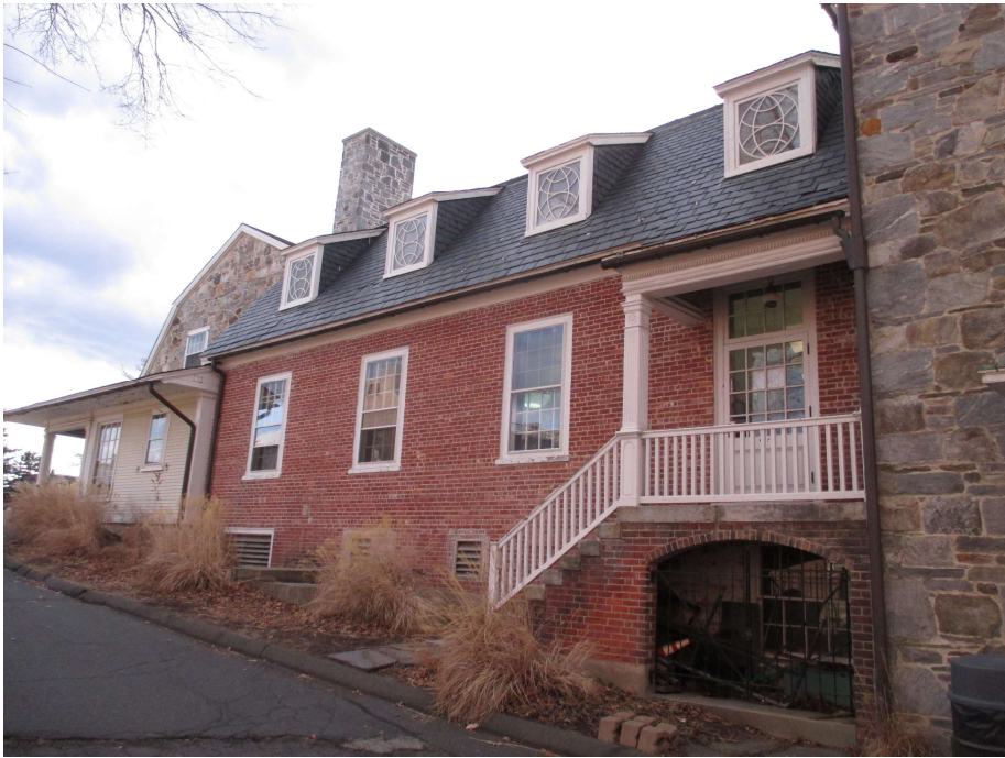
25. East elevation, view southwest
