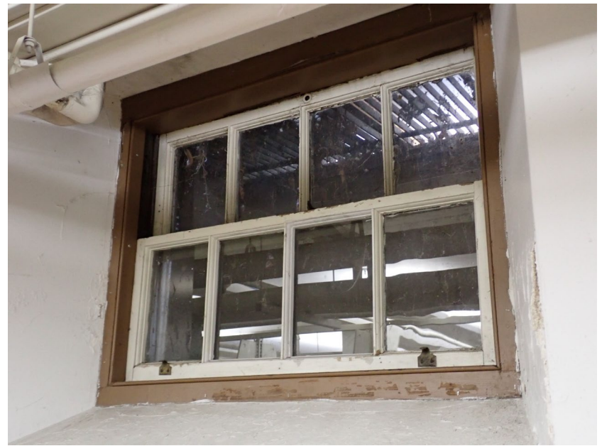
10. Basement level, south wall, typical historic double-hung wood window
