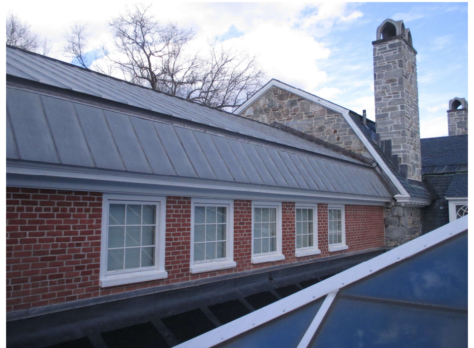
176. Roof level, view northeast
