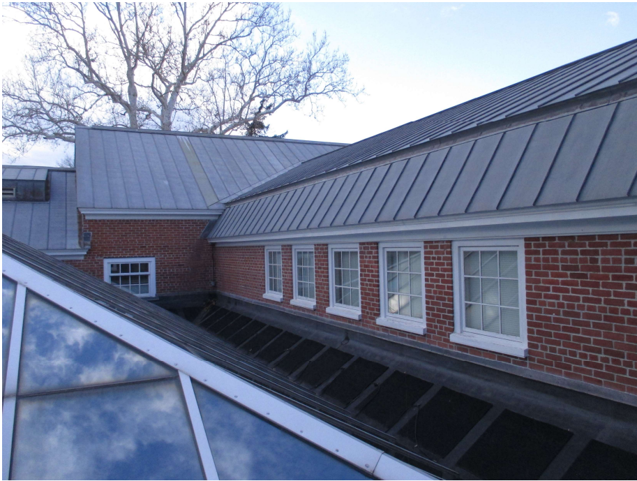
169. Roof level, view east
