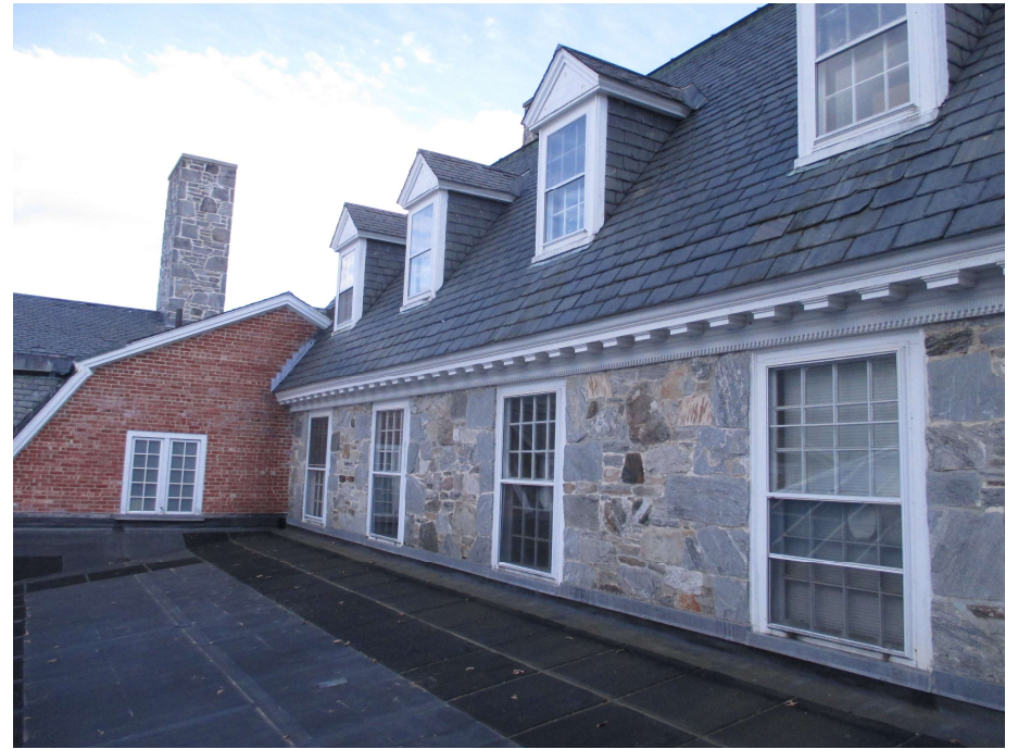
174. Roof level, view southeast
