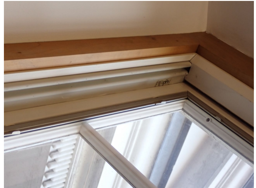
16. Basement level, north wall, detail of typical 1993 double-hung wood window condition
