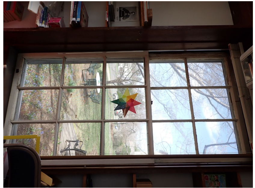
22. First floor, west wall, typical historic double-hung wood window
