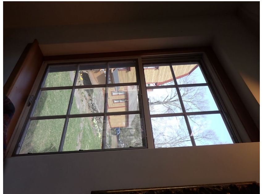
30. First floor, north wall, typical double-hung wood window at 1993 addition
