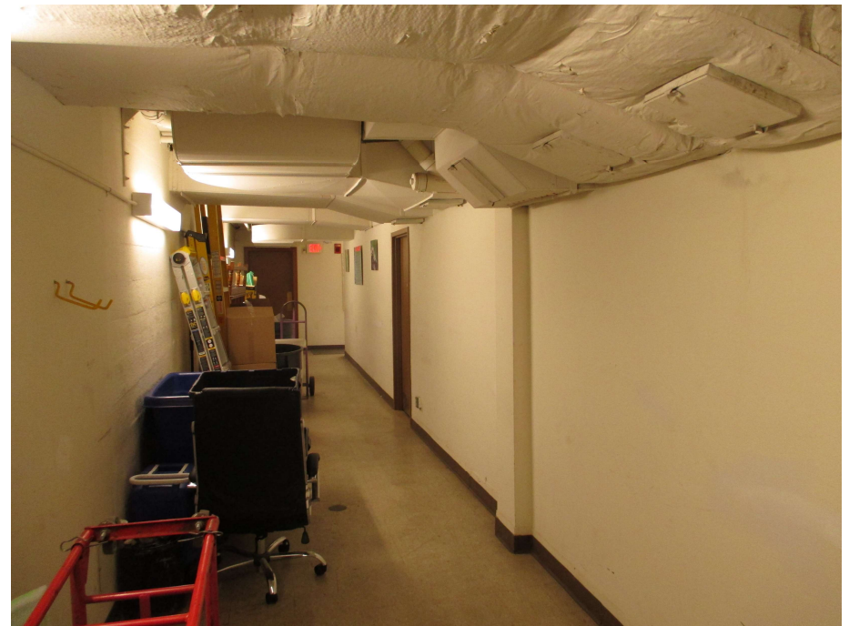
52. Lower level, corridor, view north
