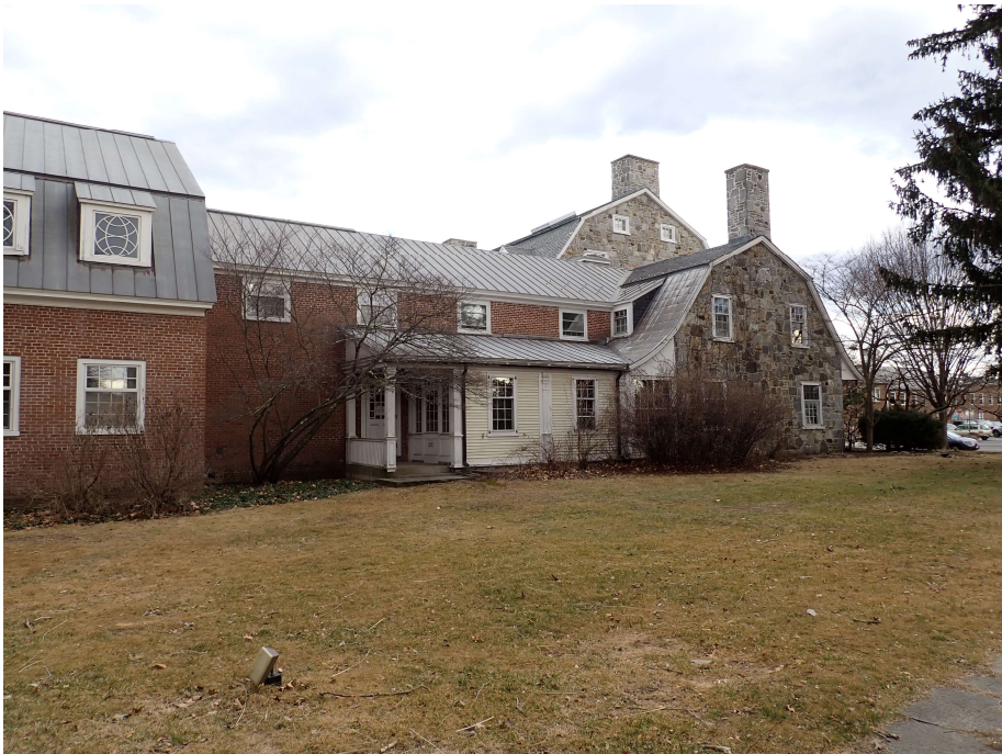
11. West elevation with 1990s addition at left, view southeast
