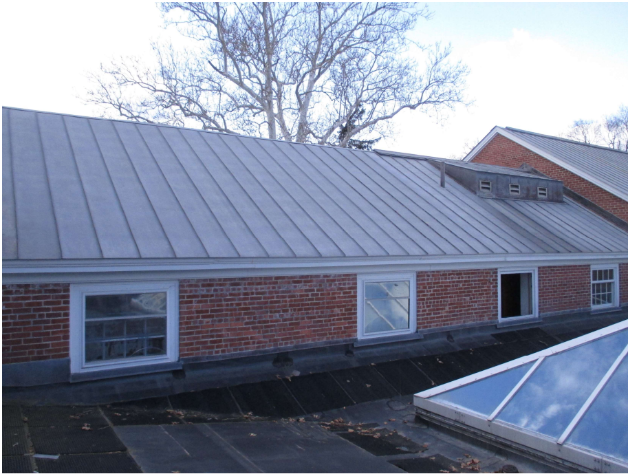
173. Roof level, view northwest
