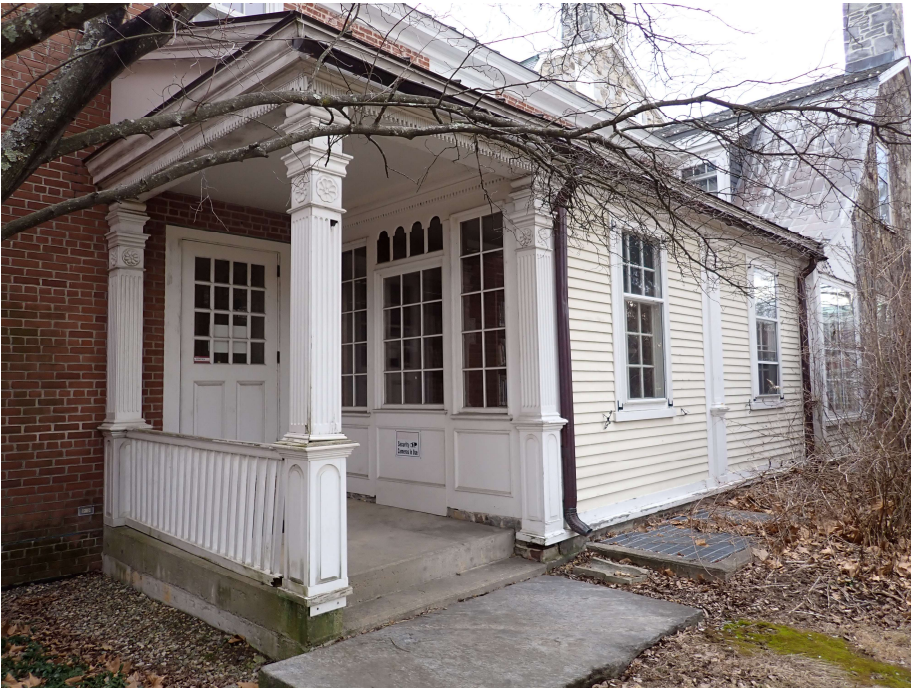
13. West elevation, secondary entrance, view southeast
