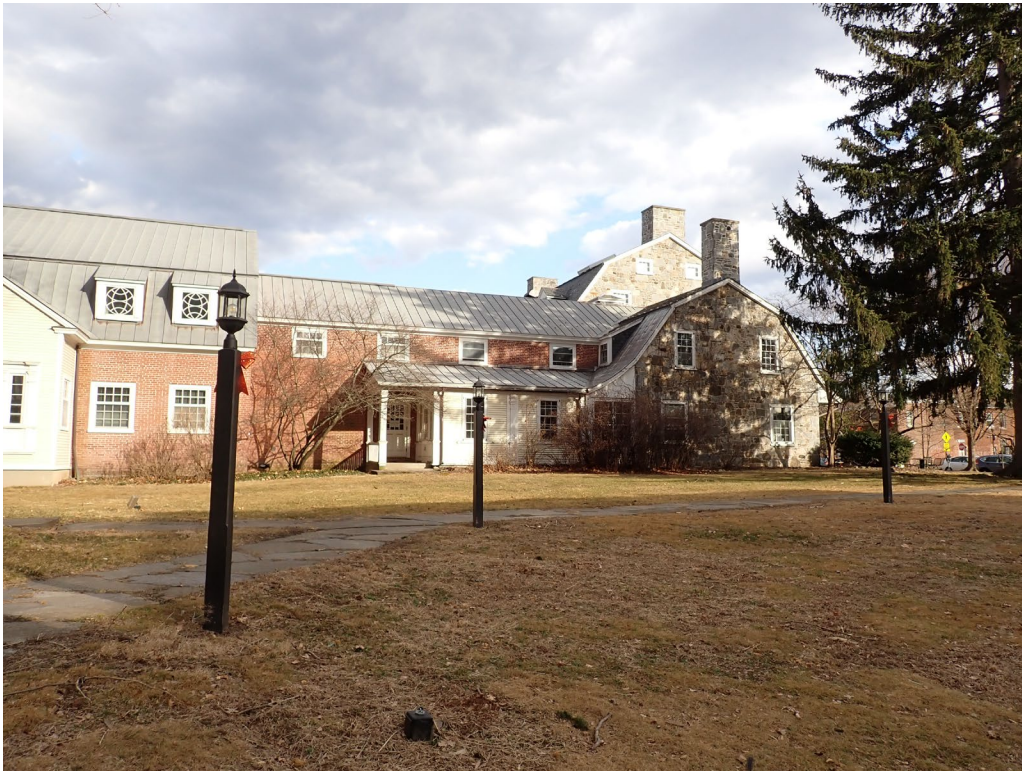
5. West elevation, view southeast
