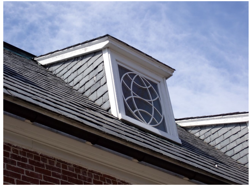
6. East elevation, typical replacement wood window at dormer
