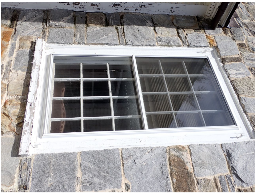
1. South elevation, first floor, typical historic double-hung wood window
