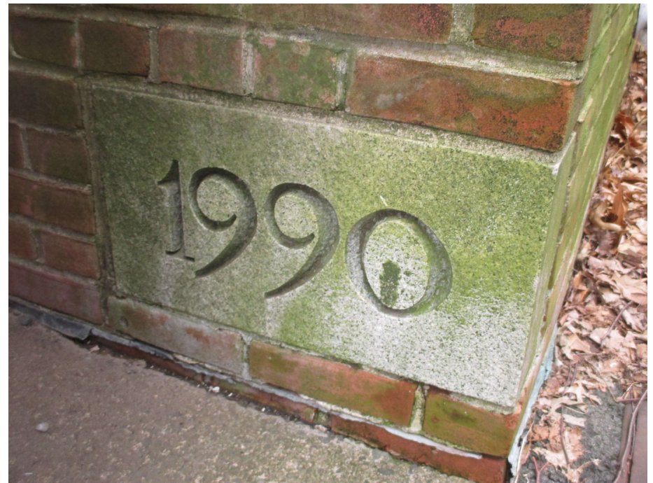
22. North elevation, cornerstone of 1990s addition, view southwest
