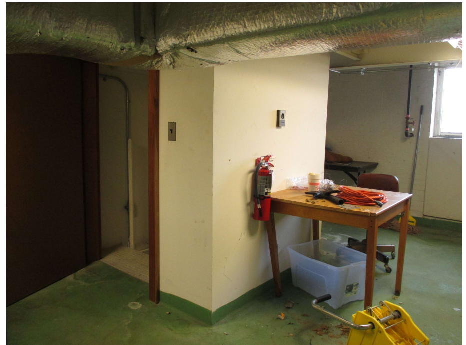
162. Third floor, mechanical room, view northeast
