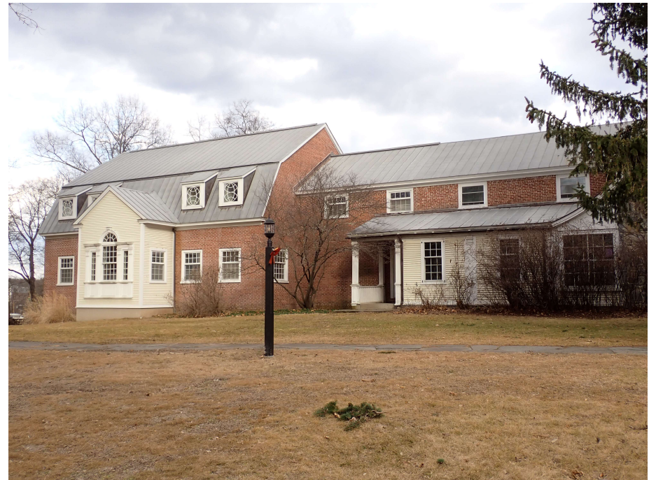
12. West elevation, 1990s additions, view northeast
