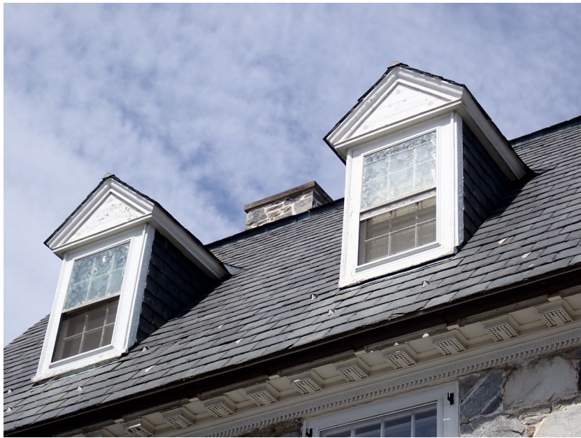
5. South elevation, typical historic double-hung wood window at dormers
