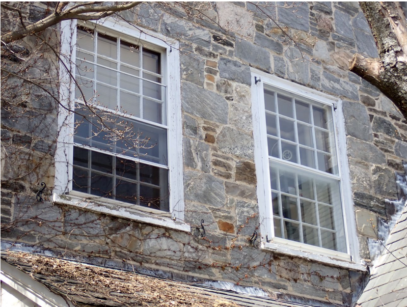
3. East elevation, second floor, typical historic double-hung wood window
