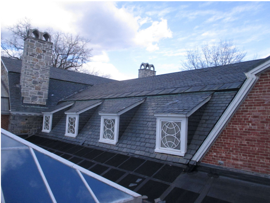
171. Roof level, view northeast
