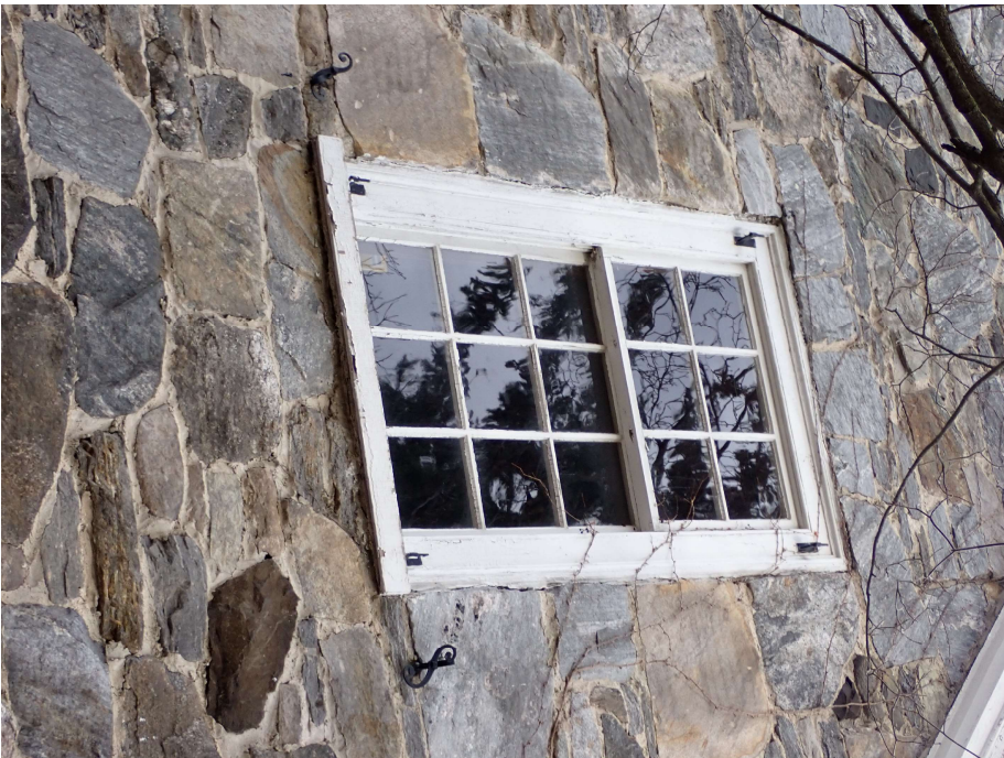
15. West elevation of west wing, typical window, view east
