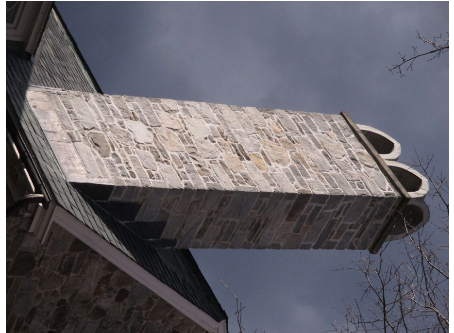
28. East elevation, chimney detail, view northwest
