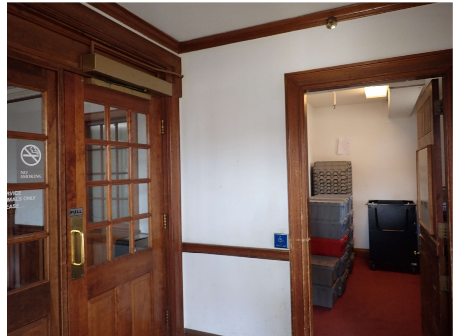
80. First floor, southeast entry vestibule, view northwest
