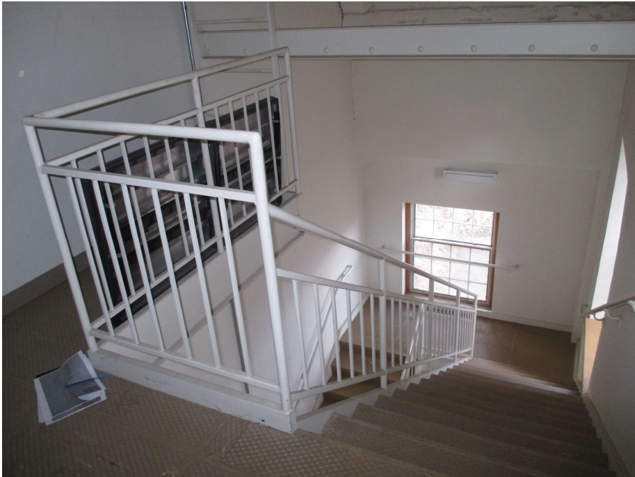
143. Second floor, northeast stair, view northwest
