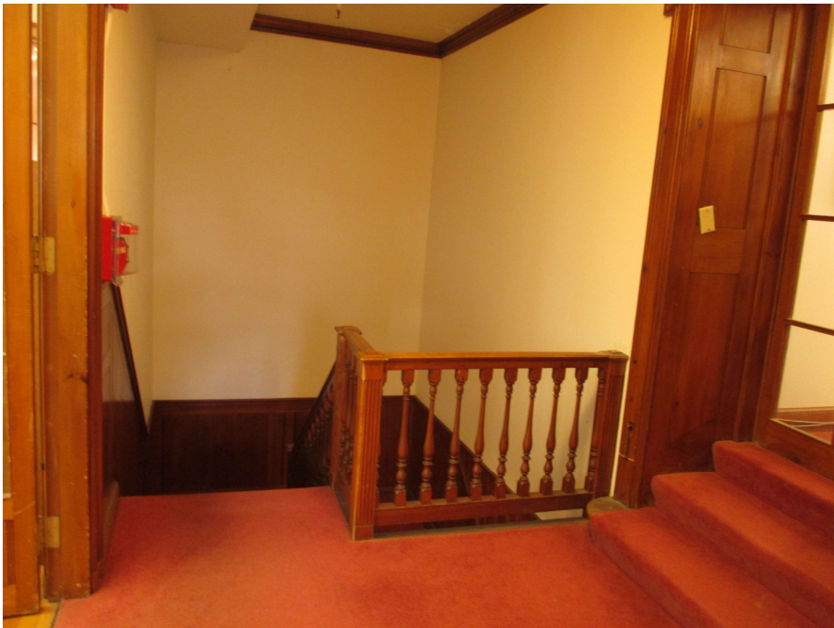
127. Second floor, southwest stair, view northeast
