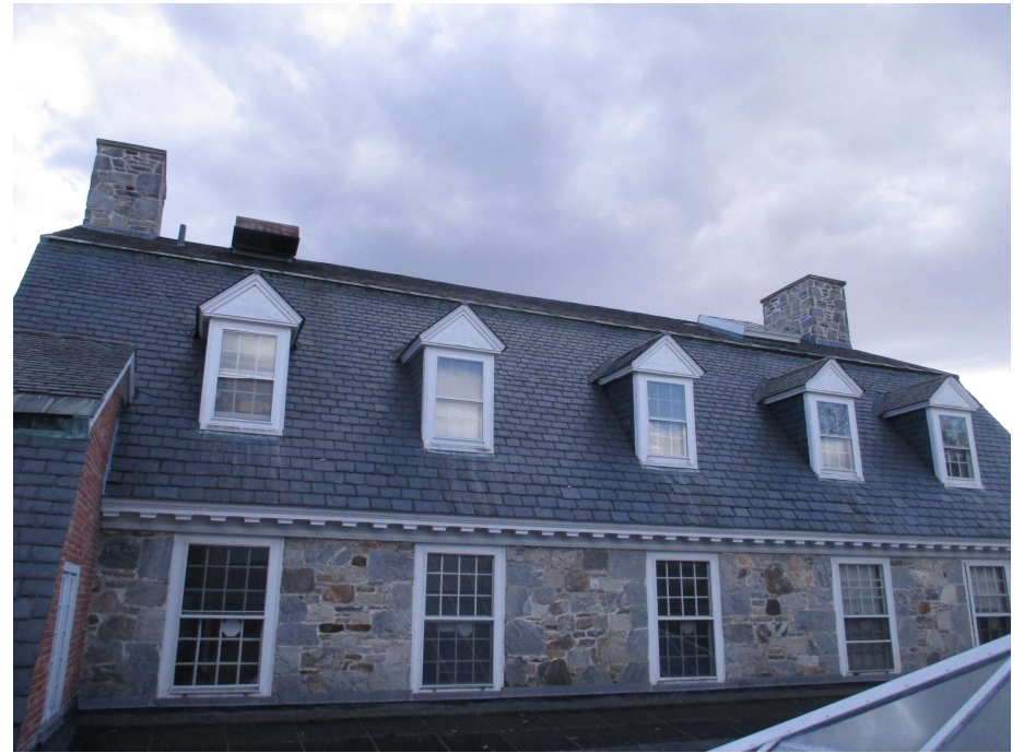
170. Roof level, view south
