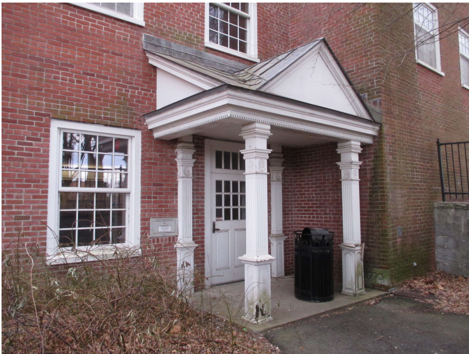
21. North elevation, secondary entrance, view southwest
