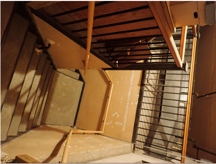
165. Attic level, main stair, view south
