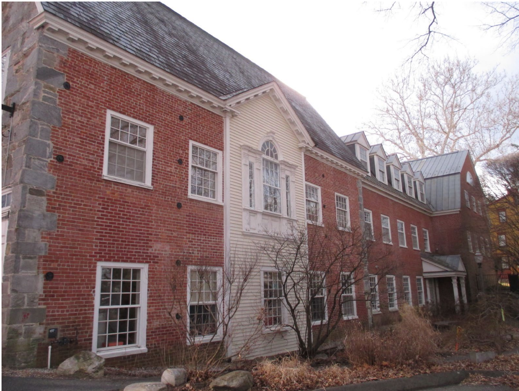
3. North elevation, view southwest
