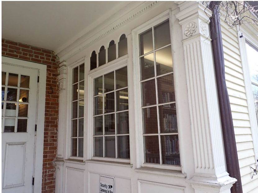
7. West elevation, first floor, typical replacement wood window
