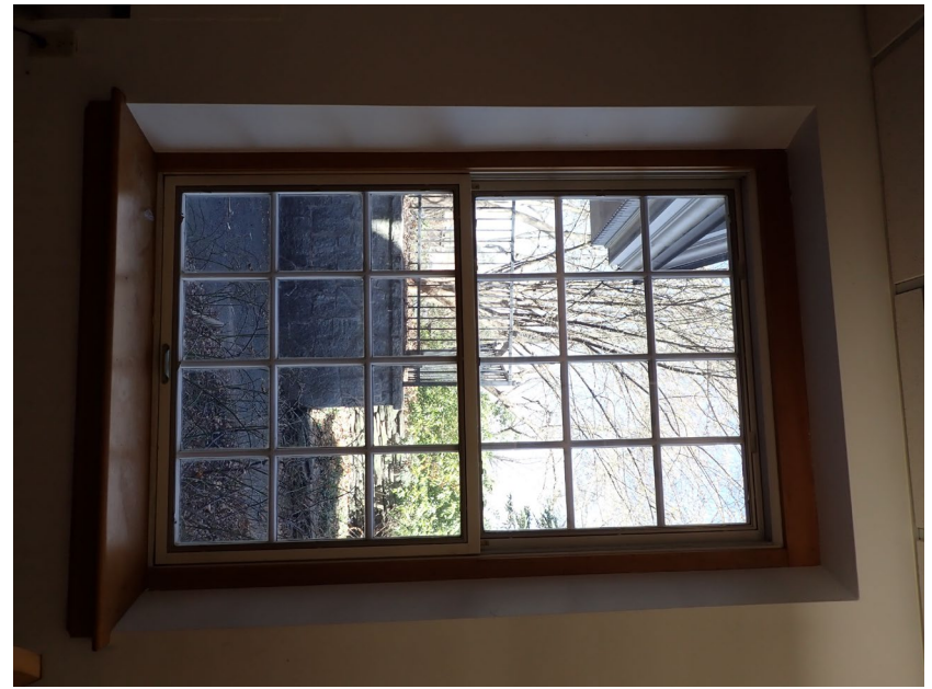
14. Basement level, north wall, typical double-hung wood window at 1993 addition
