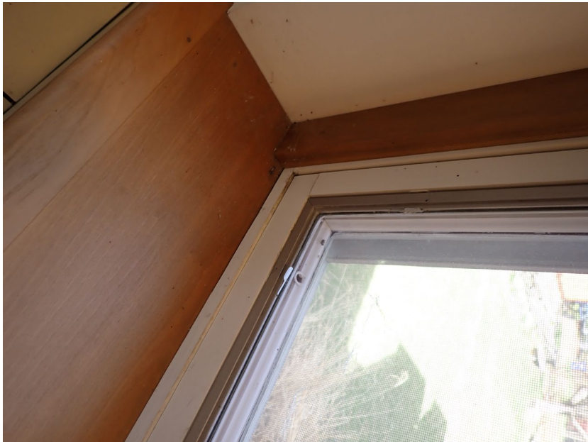
31. First floor, north wall, detail of typical 1993 wood window condition
