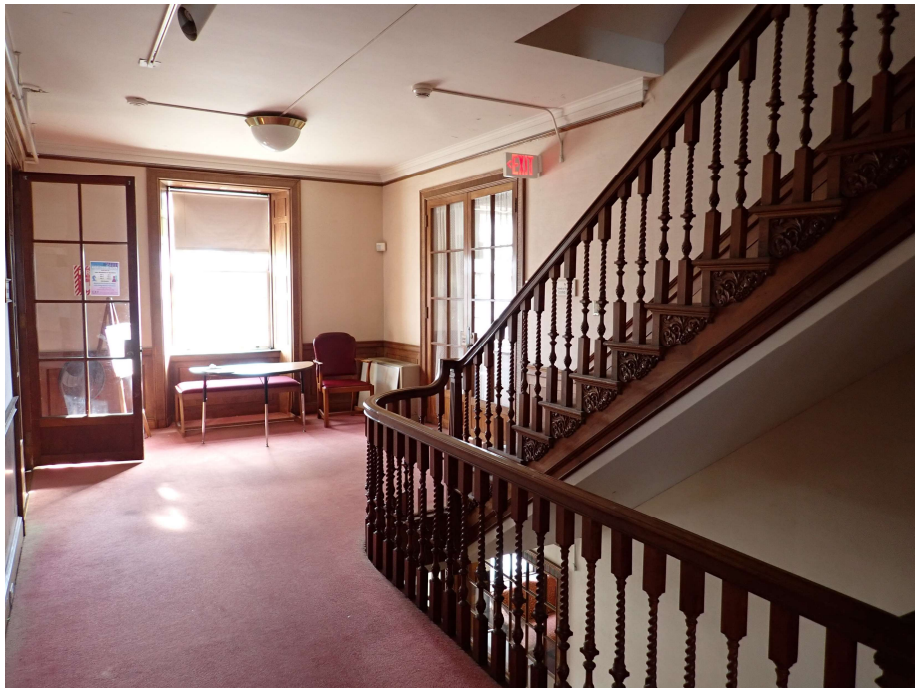
119. Second floor, main stair hall, view southwest
