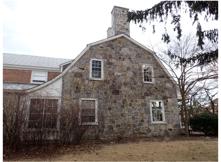
10. West elevation of west wing, view east
