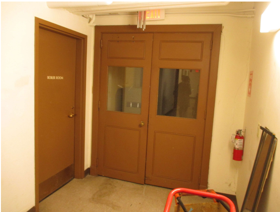
51. Lower level, entry doors to mechanical area, view southeast
