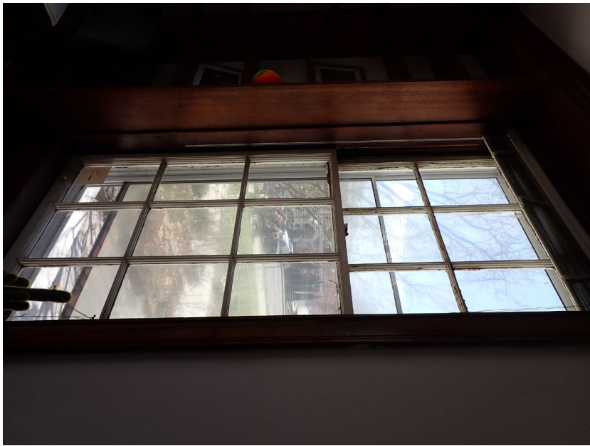
17. First floor, south wall, typical historic double-hung wood window
