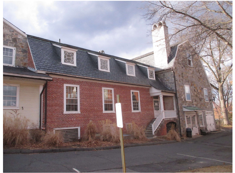
26. East elevation, view northwest
